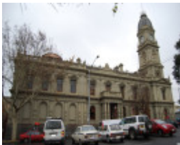
3016 Hotham Town Hall Queensberry St View 02
