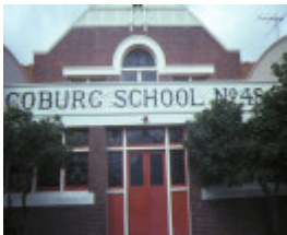
infant building & shelter shed coburg primary school no 484 bell street coburg entrance sep 84
