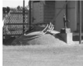
Domed cement rendered brick underground tank, with iron handpump.
