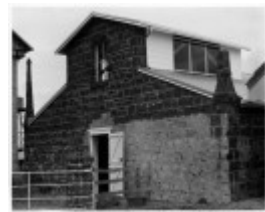
Warrawong Shearing Shed
