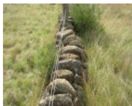
Dry Stone Wall K164 - Eastern Boundary
