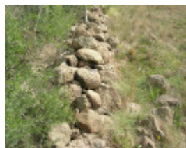
Dry Stone Wall K166 - south boundary
