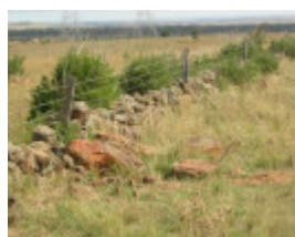
Dry Stone Wall K165 - north boundary
