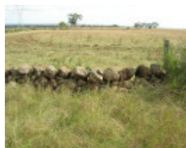
Dry Stone Wall K164 - Eastern Boundary
