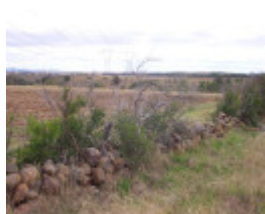
Dry Stone Wall K165 - north boundary
