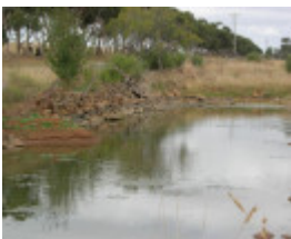
Dry Stone Wall K159 - eastern boundary
