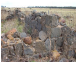
Ruins of the rubble bluestone house
