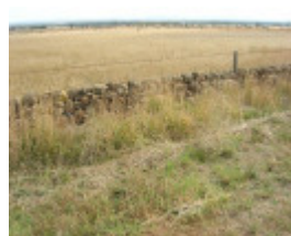
Dry Stone Wall K159 - eastern boundary
