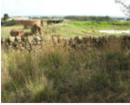
Dry Stone Wall K159 - eastern boundary
