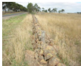
Dry Stone Wall K159 - eastern boundary
