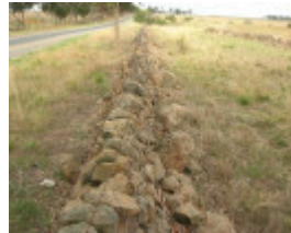
Dry Stone Wall K159 - eastern boundary
