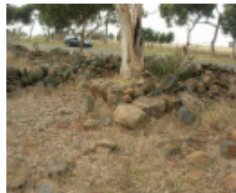
Dry Stone Wall K159 - eastern boundary
