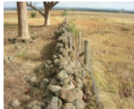
Dry Stone Wall K158 - northern boundary
