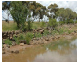
Dry Stone Wall K172 - Sheep Wash
