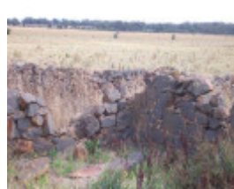
The ruins of the rubble bluestone house
