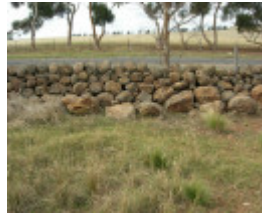
Dry Stone Wall K159 - eastern boundary
