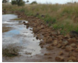
Dry Stone Wall K172 - Sheep Wash
