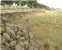
Dry Stone Wall K159 - eastern boundary
