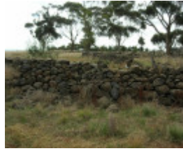
Dry Stone Wall K161 - Internal Stock Holding Yard
