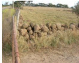
Dry Stone Wall F181 - western boundary
