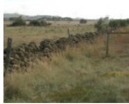
Dry Stone Wall F181 - western boundary
