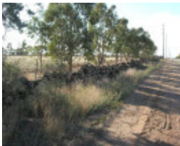
Dry Stone Wall F186 - southern boundary
