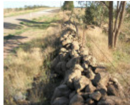
Dry Stone Wall F186 - southern boundary
