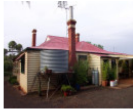
Rear elevation of house
