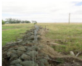
Dry Stone Wall B129 - northern boundary
