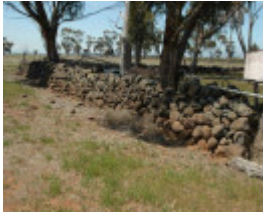
Dry Stone Wall B74
