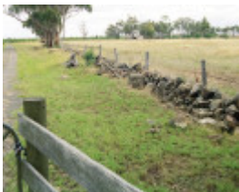
Dry Stone Wall B128 - southern boundary
