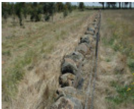
Dry Stone Wall B76
