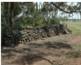
Dry Stone Wall B28
