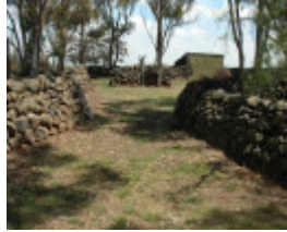
Dry Stone Wall B75
