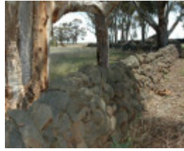
Dry Stone Wall B75
