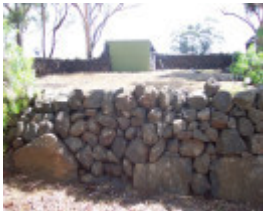
Dry stone wall stock yard
