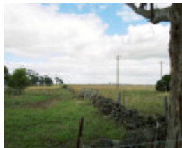
Dry Stone Wall B129 - northern boundary
