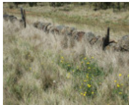
Dry Stone Wall B76
