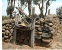
Dry Stone Wall B75
