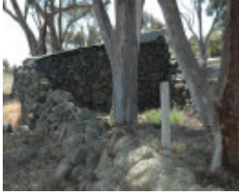
Dry Stone Wall B75
