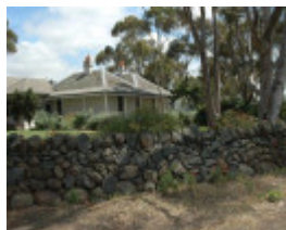
Dry Stone Wall B28
