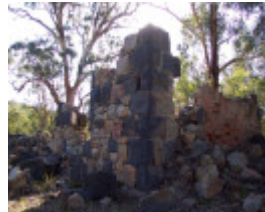
Ruin, thought to be the Greenhills Station Shearers' Quarters
