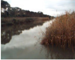
Koo Wee Rup Swamp drains & Bridges
