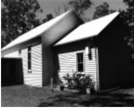
Pakenham Upper Civic & Residential Precinct & Upper hall
