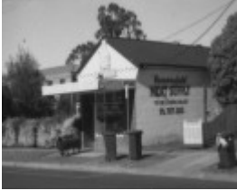
Wood Street Commercial & Civic Precinct
