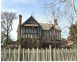
2 Ash Grove, Malvern East
