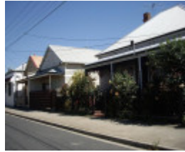
HO15(4) - Yarraville residential heritage area.JPG
