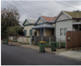
HO15(1) - Yarraville Residential Heritage Area.JPG
