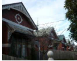
Fenton Street north side
