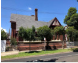
9-23 Densham Road, Armada
