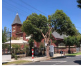
9-23 Densham Road, Armada
