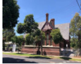
9-23 Densham Road, Armada
