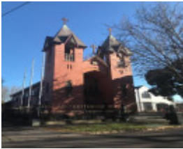
3B Epping Street, Malvern East
