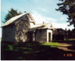
Dollar State School No. 3473 (former)
