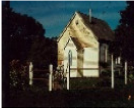
Dumbalk North Methodist Church (former)
