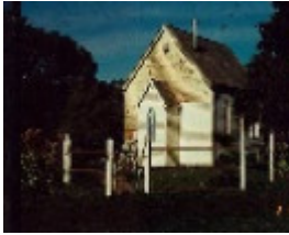
Dumbalk North Methodist Church (former)
