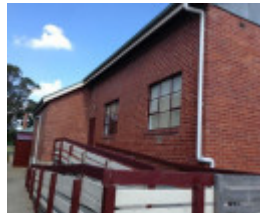
Fish Creek Memorial Hall 1959 Supper Room addition
