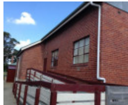
Fish Creek Memorial Hall 1959 Supper Room addition
