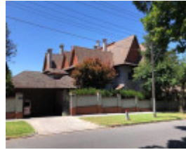
224 Kooyong Road, Toorak
