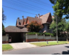
224 Kooyong Road, Toorak
