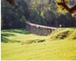
Three Railway Bridges
