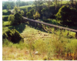
Three Railway Bridges
