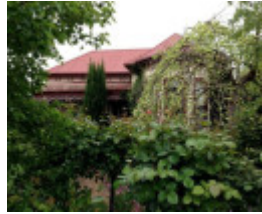
House 23 Bridge Street
