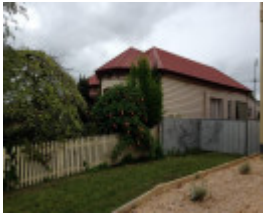
House 23 Bridge Street
