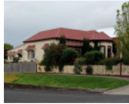
House 23 Bridge Street
