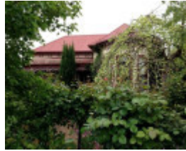
House 23 Bridge Street
