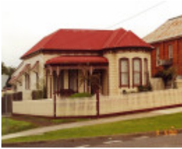
Dwelling at 23 Bridge Street Korumburra 3950
