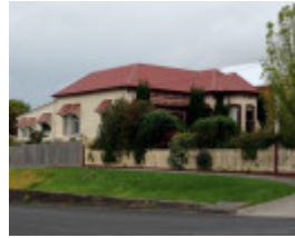
House 23 Bridge Street
