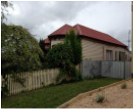
House 23 Bridge Street
