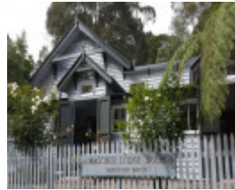
Former Kilcunda Road State School
