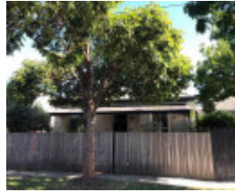
66-72 Peel Street, Windsor
