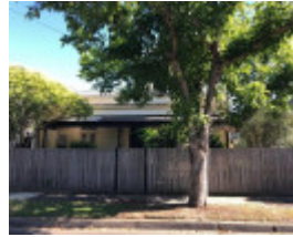
66-72 Peel Street, Windsor
