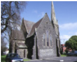
1 holy trinity anglican church complex sydney road coburg side view of church aug1992
