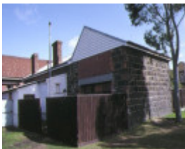
holy trinity anglican church complex sydney road coburg school rear view aug1992
