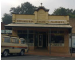
Falconer Building (former, 2020)
