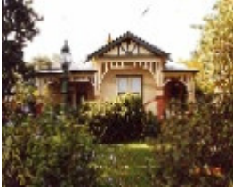
Dwelling at 20 Victoria Street Korumburra 3950
