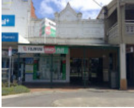
Shops, 8-10 Bair Street (2020)
