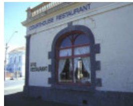
former adam reas store colac detail side window feb1985
