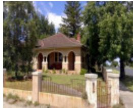
Former UV Knight's House, 26 Ogilvy St
