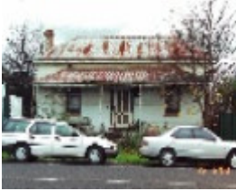
Dwelling AT 10 Roughead Street Leongatha 3953
