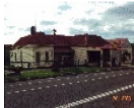
Former Bigelow's Store
