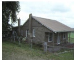
yeringberg maroondah hwy coldstream cottage view dec1987
