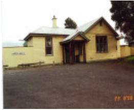
Mirboo North Railway Station (former)
