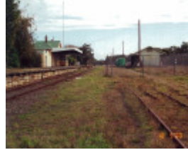
Nyora Railway Station complex
