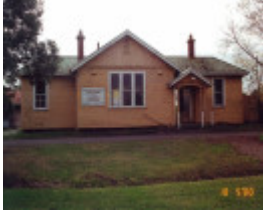
Nyora Railway Station complex
