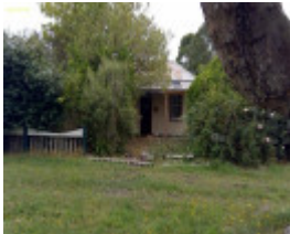
Butter Factory Manager's Residence (former, 2020)
