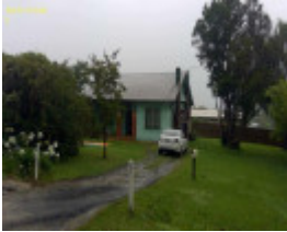
Toora Butter Factory Manager's Residence (former)
