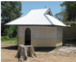
AUBURN PRIMARY SCHOOL NO.2948 SOHE 2008
