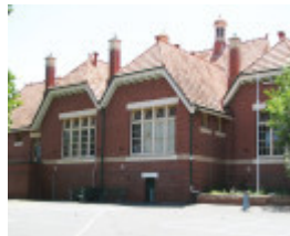
AUBURN PRIMARY SCHOOL NO.2948 SOHE 2008
