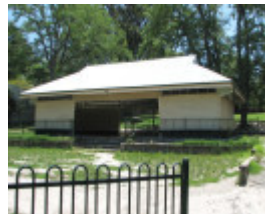
AUBURN PRIMARY SCHOOL NO.2948 SOHE 2008
