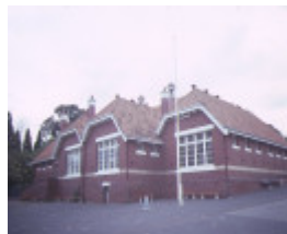
auburn primary school no 2948 rear view
