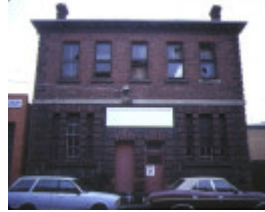
former grosvenor common school bond street collingwood front view jun1985
