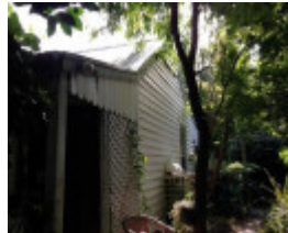
South side elevation of north cottage
