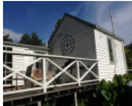
Formerly detached rear kitchen (now bathroom)
