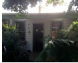
Entrance to north cottage
