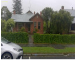
Toora Post Office Residence
