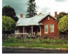
Toora Post Office residence (2000)
