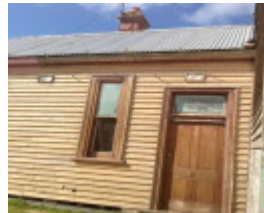
North side doorway
