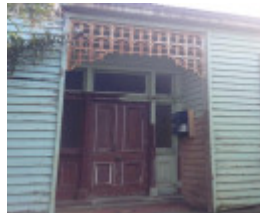
Residential entrance on south side
