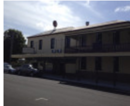
Royal Standard Hotel, showing 1939 additions at left (2015)
