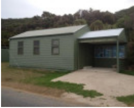
Walkerville North Public Hall
