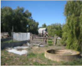
Bael Bael Homestead Bael Bael 10 Sept 2008 mz Water Tank and Stock Yard
