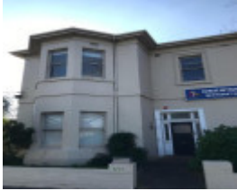
1219-1225 Dandenong Road, Malvern East
