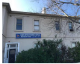
1219-1225 Dandenong Road, Malvern East
