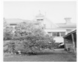
A 1975 photograph of the rear of Aldene showing the outbuilding in the foreground.
