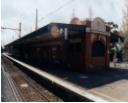
HEIDELBERG RAILWAY STATION
